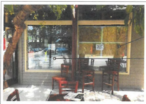
Existing Windows (from Perry St)
