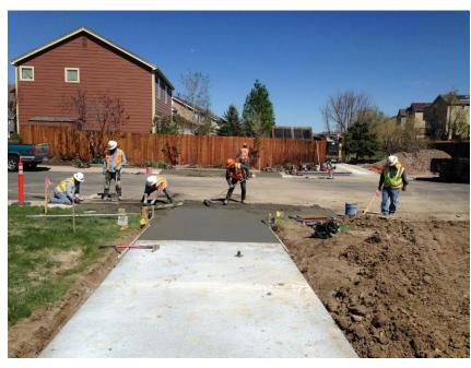
In May, the contractor completed the last remaining 250-linear feet of trail, installed four ADA accessible ramps, finalized backfill and cleared and grubbed the Tabor Court connection to prepare for wall construction. In addition, 310-linear feet of railing was manufactured to be installed in June. Restoration of impacted areas will begin once the railing is installed.
