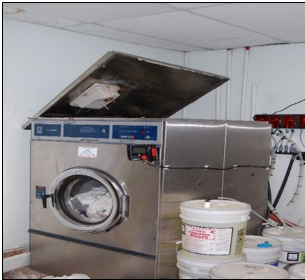
Dryer where a fire originated
