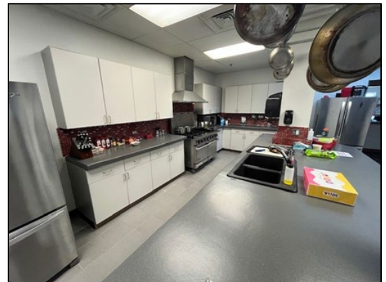
Station 154 counter top refinish
