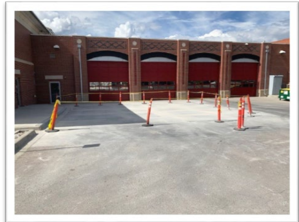
Station 151 Rear Pad Repair
