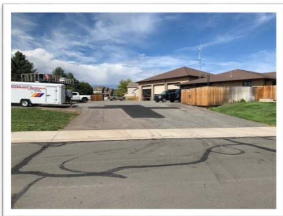
Station 153 Rear Drive Repair
