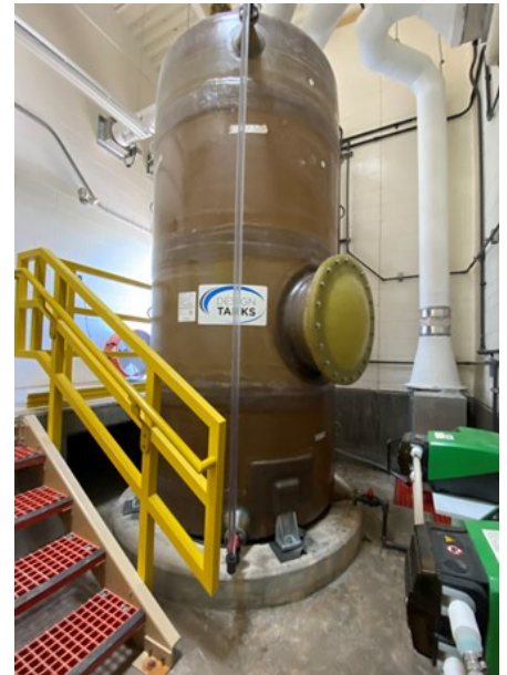
Newly installed Hypo tank
