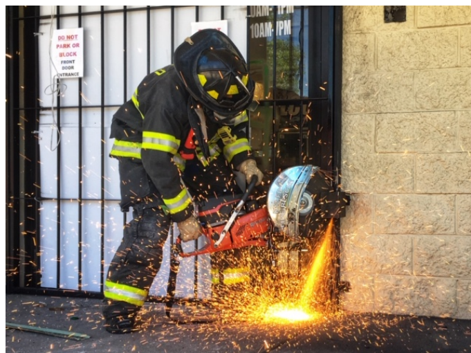
forcible entry saw work
