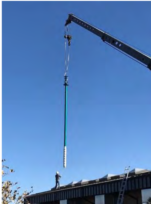
Green Zone Pump Replacement at the RWRWTC
