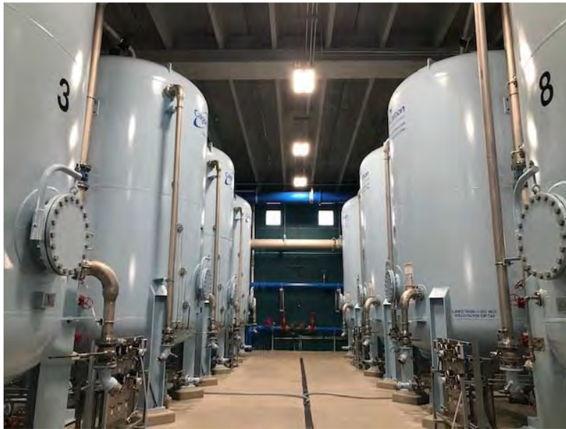
Advanced Treatment GAC filters at the PCWPF
