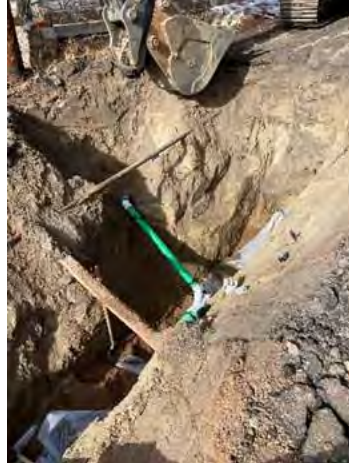
Water and sewer main replacement in the Craig and Gould neighborhood.
