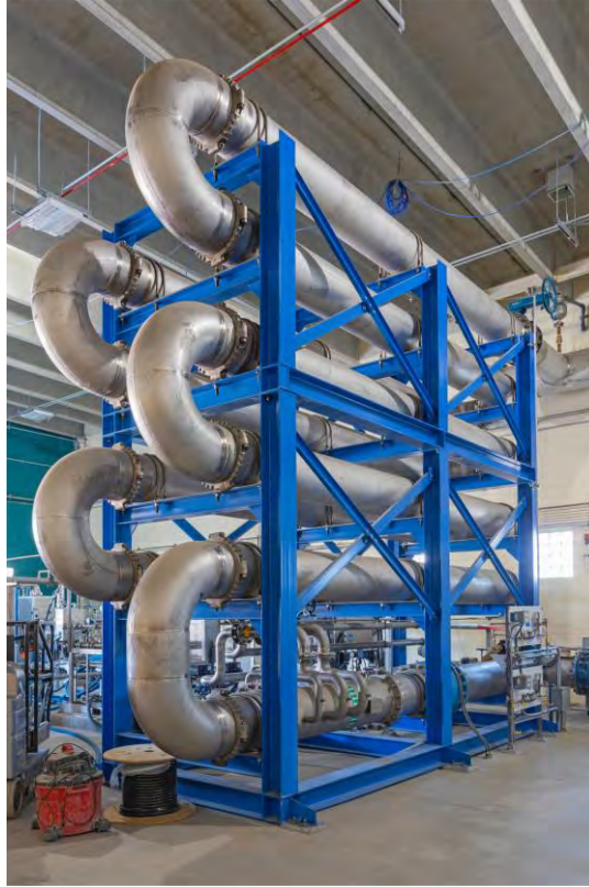
Advanced Treatment Ozone Contact Time Piping at the PCWPF
