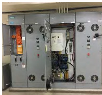
Upgraded Crystal Valley Pump Station Motor Control Center (MCC) and VFDs
