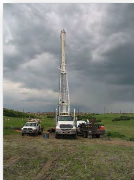
Rig set up over existing well to pull down-hole equipment.
