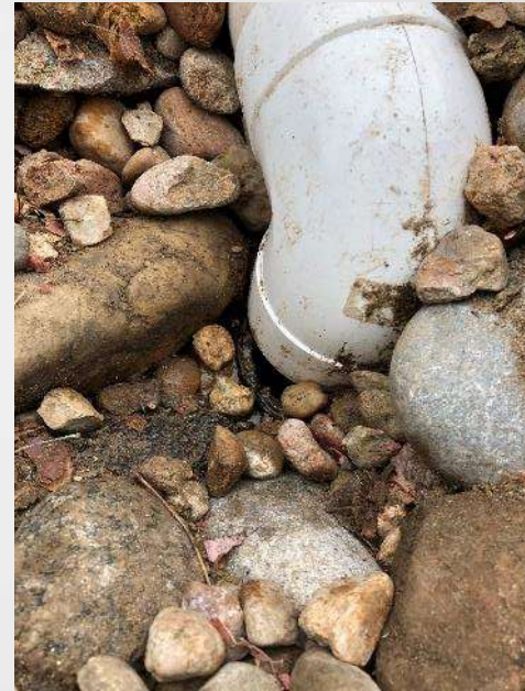
Example of resident removing an inlet grate to connect a private pipe to underdrain
