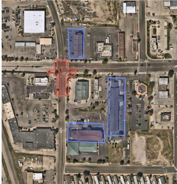
Wolfensberger Rd. & Park St. Intersection Improvements
