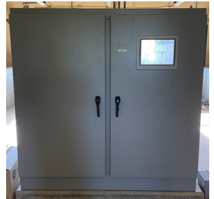
New PLC cabinets with PanelView screens
