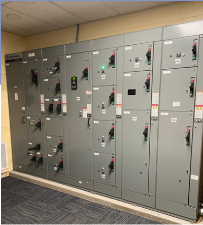
New Motor Control Center and Programmable Logic Controller
