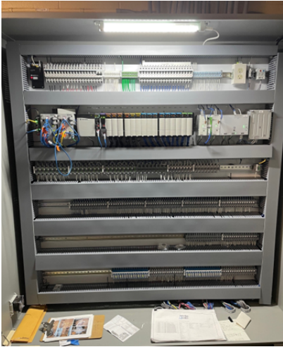
New Motor Control Center and Programmable Logic Controller
