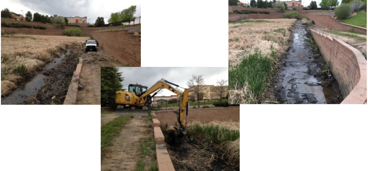
The Stormwater Team conducted maintenance of the stormwater pond located near the KinderCare at Founders and Front St. A total of 110 cubic yards of material were removed, restoring the trickle channel!
