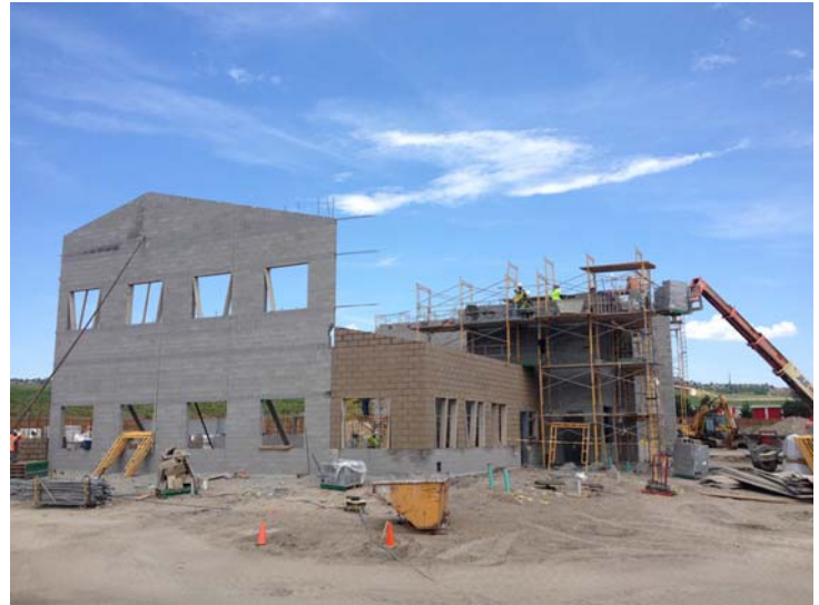
Installation of concrete masonry units
