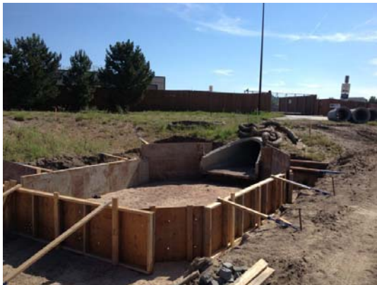
Formwork for new concrete forebay
