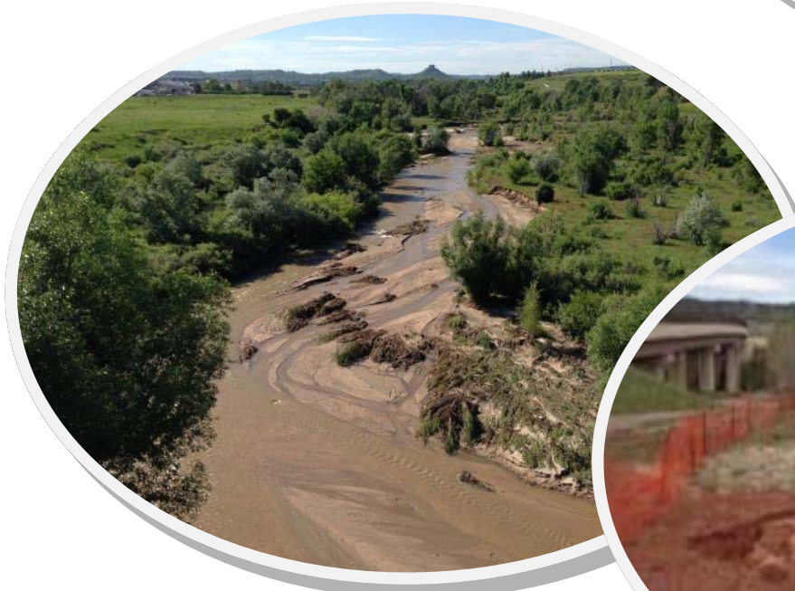
E. Plum Creek and N. Meadows bridge
