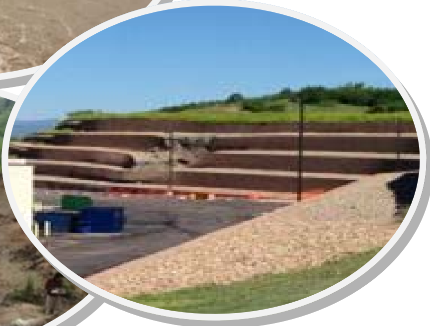
Retaining wall behind Sprouts
