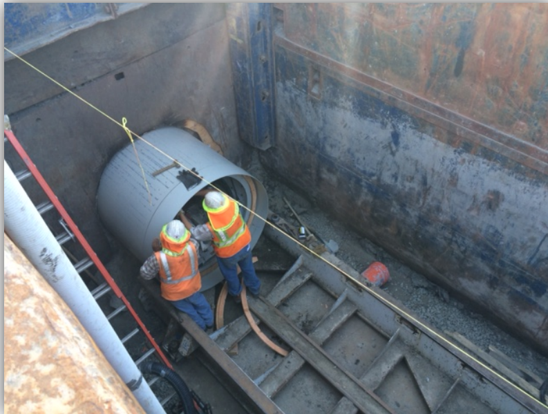
JACKED PIPE UNDER UNION PACIFIC RAILROAD
