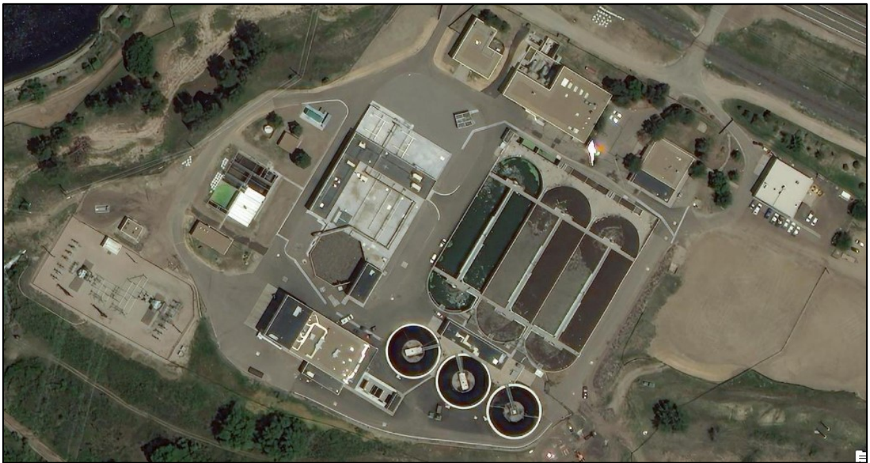
Figure 14: Aerial View of the Plum Creek Water Reclamation Authority Facility (CRWA)
