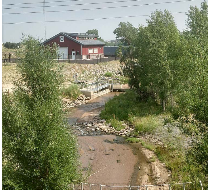
Figure 9: Town of Castle Rock's Plum Creek Diversion
