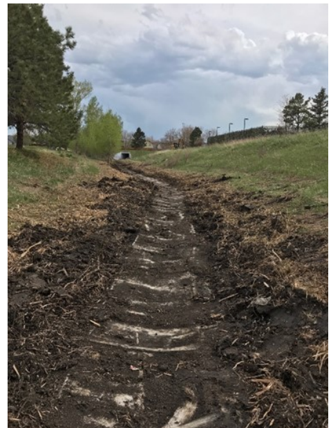
The Stormwater Team restored the trickle channel near Founders Park
