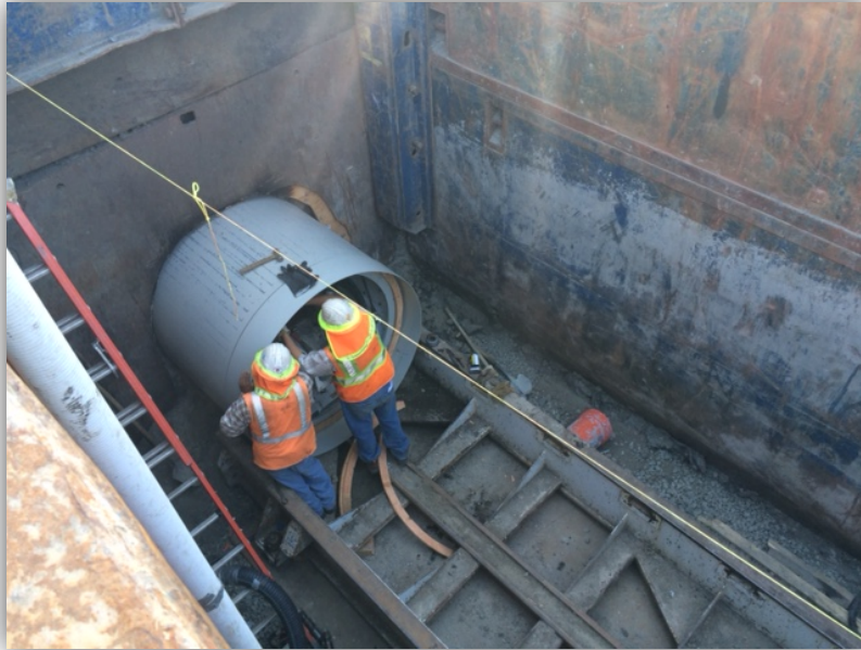
JACKED PIPE UNDER UNION PACIFIC RAILROAD
