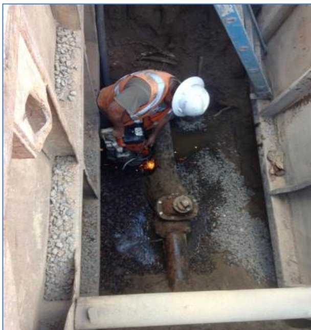
Cutting valve out of system to install new valve
