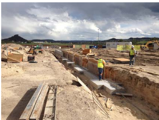
Installation of concrete foundation footings and stemwalls
