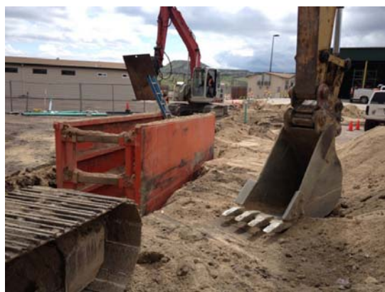
Installation of new sanitary sewer service line to the building
