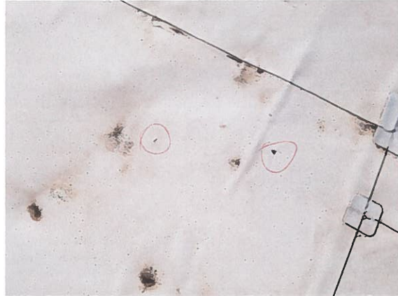
Photo #44: Holes in roof membrane. There are several on this roof level.
