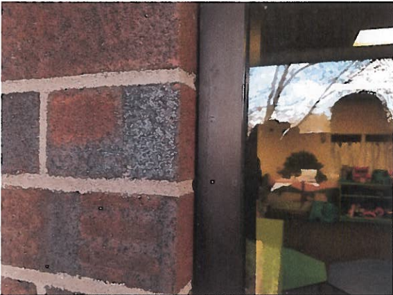
Photo #3: No caulking around window.
