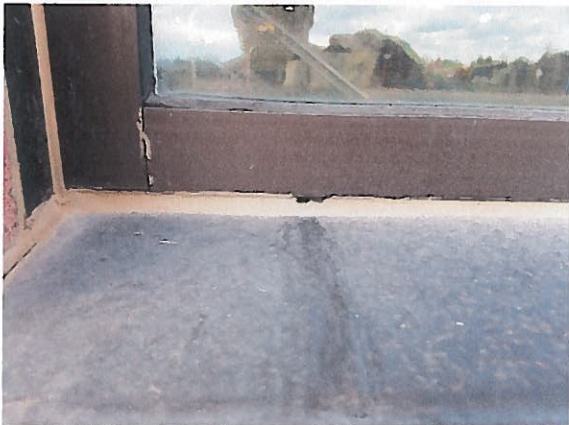
Photo #27: Newer sealant at window with properly exposed weep holes.
