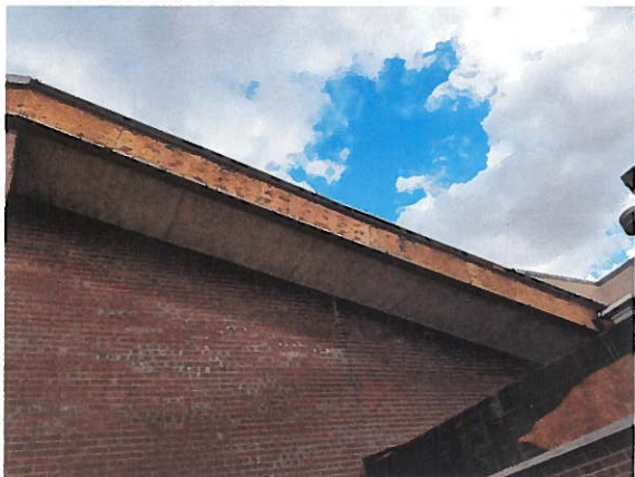
Photo #16: Water damage in exposed tectum soffit.
