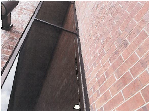
Photo #19: Failed caulking.
