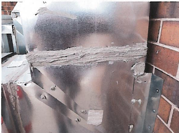
Photo #9: Joints in metal duct work could be sealed with peel & stick tape.
