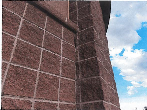
Photo #26: Damage at wall to wall joint.
