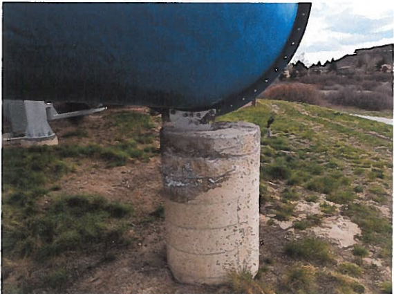
Photo #23: Posts should be waterproofed to avoid further damage.
