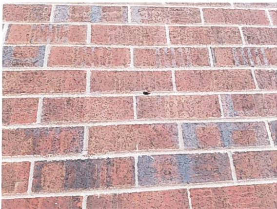
Photo #34: Hole in mortar should be repaired.
