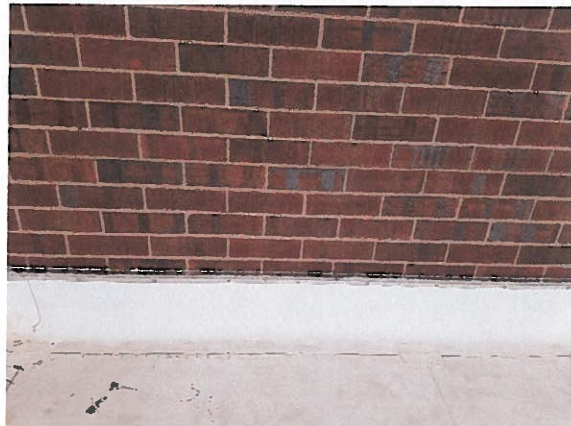
Photo #52: Term bar only, no counter flashing.
