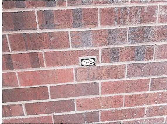
Photo #2: Missing electric cover .
