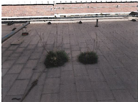
Photo #47: Drains blocked by growth.
