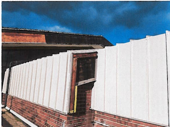
Photo #48: Panel missing at corner. Roofing contractor states that this is not in current scope of work.
