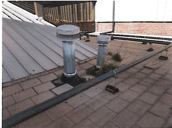
Photo #46: Grass and weeds growing throughout this roof area.
