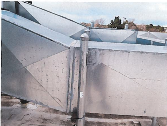
Photo #53: Metal duct work. Seams should be sealed.
