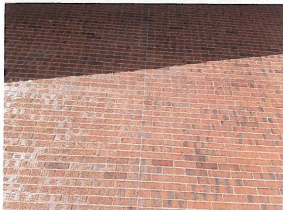
Photo #30: Joint starting to fail.
