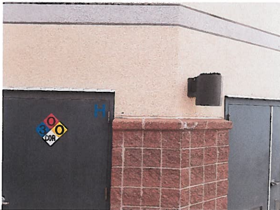
Photo #21: Efflorescence from water entry.
