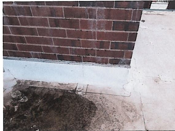
Photo #38: In discussion with roofing contractor, they acknowledge that they used the basic details as required to meet warranty. No counter flashing.
