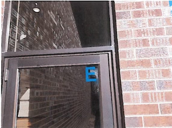
Photo #31: Failed sealant.
