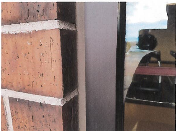
Photo #11: Properly sealed window to wall joint.
