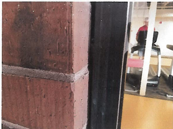
Photo #10: No caulking in windows in front of exercise room.
