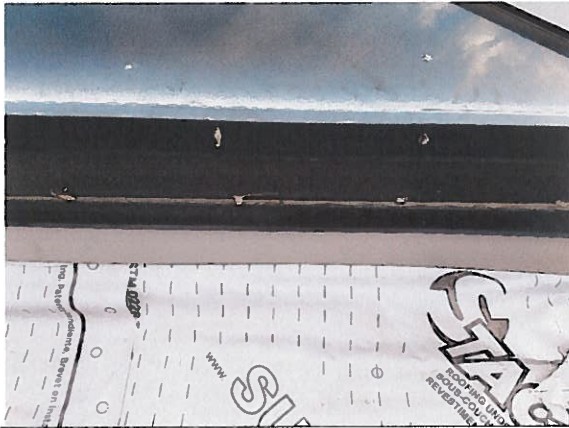
Photo #55: Weep holes blocked n skylight.
