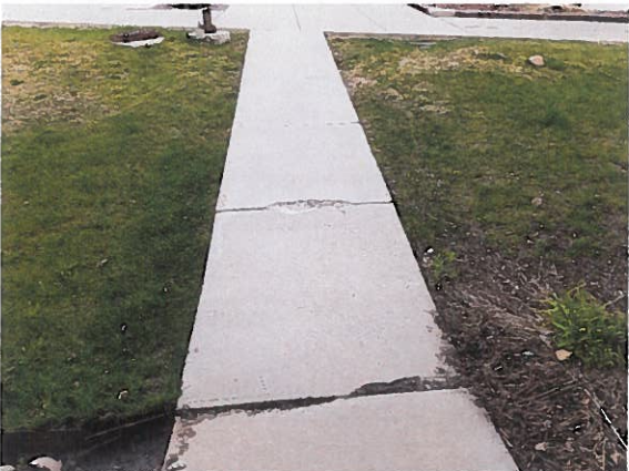
Photo #5: Damage walk way is a trip hazard.
