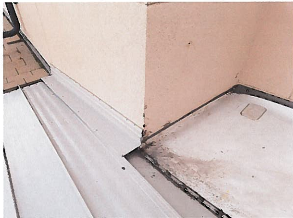
Photo #45: Damage to EIFS wall at lower roof tie in.
