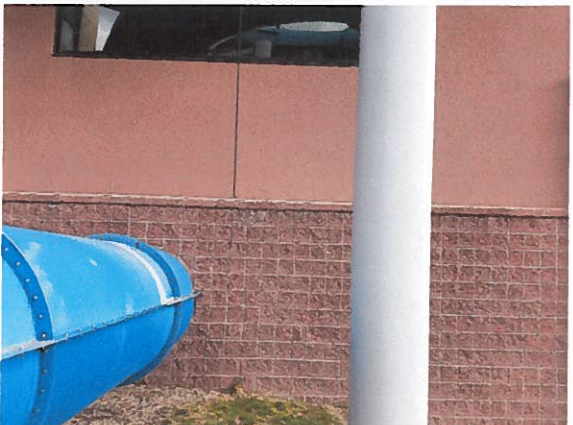
Photo #24: Water damage below caulk joint. Seal at slide entry to wall should be waterproofed.
