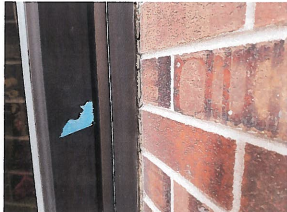
Photo #20: Failed caulking.
