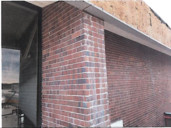
Photo #37: On roof at top of ladder, damage to wall from water entry from roof above.
