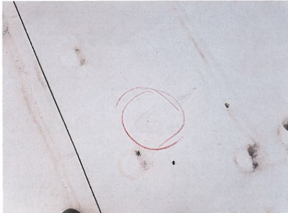
Photo #43: Higher circular roof. Hole in membrane.
