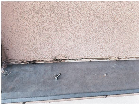
Photo #57: Joint the length of counter flashing is failed.
