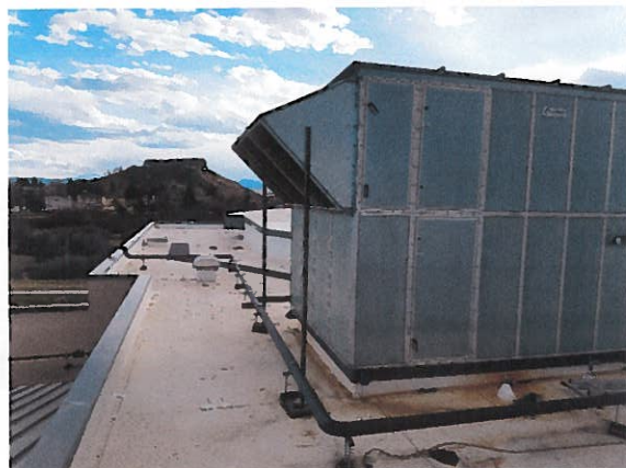
Photo #39: Roof with large roof top air handler for pool.
