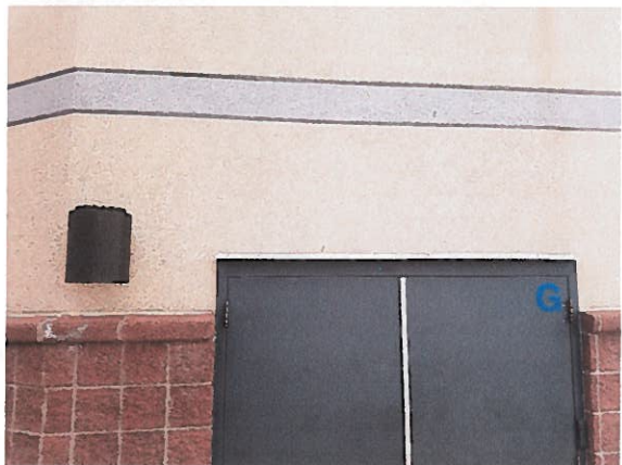
Photo #22: Efflorescence.
