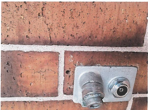
Photo #12: Drilled hole in brick should be sealed.
