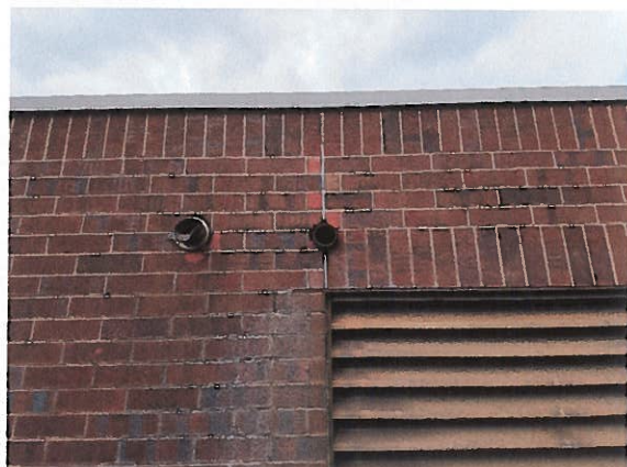
Photo #28: Water drain pipes from roof above are too short and water is damaging wall.
