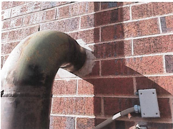
Photo #29: Some pipes through wall are properly sealed while others are not.
