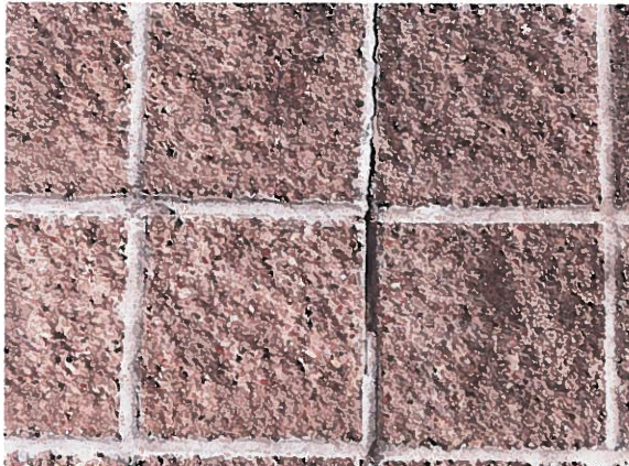
Photo #25: Damage to wall joints should be repaired.
