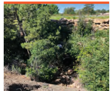
Boulder retaining wall adjacent to Prairie Hawk Drive.
