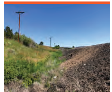
Ditch between BNSF and Prairie Hawk Drive.
