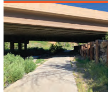
Existing retaining wall upstream of I-25 Bridge over East Plum Creek.
