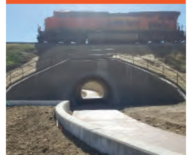
The Fossil Creek Pedestrian Tunnel (Lithos staff experience) spans 70 linear feet underneath BNSF.
