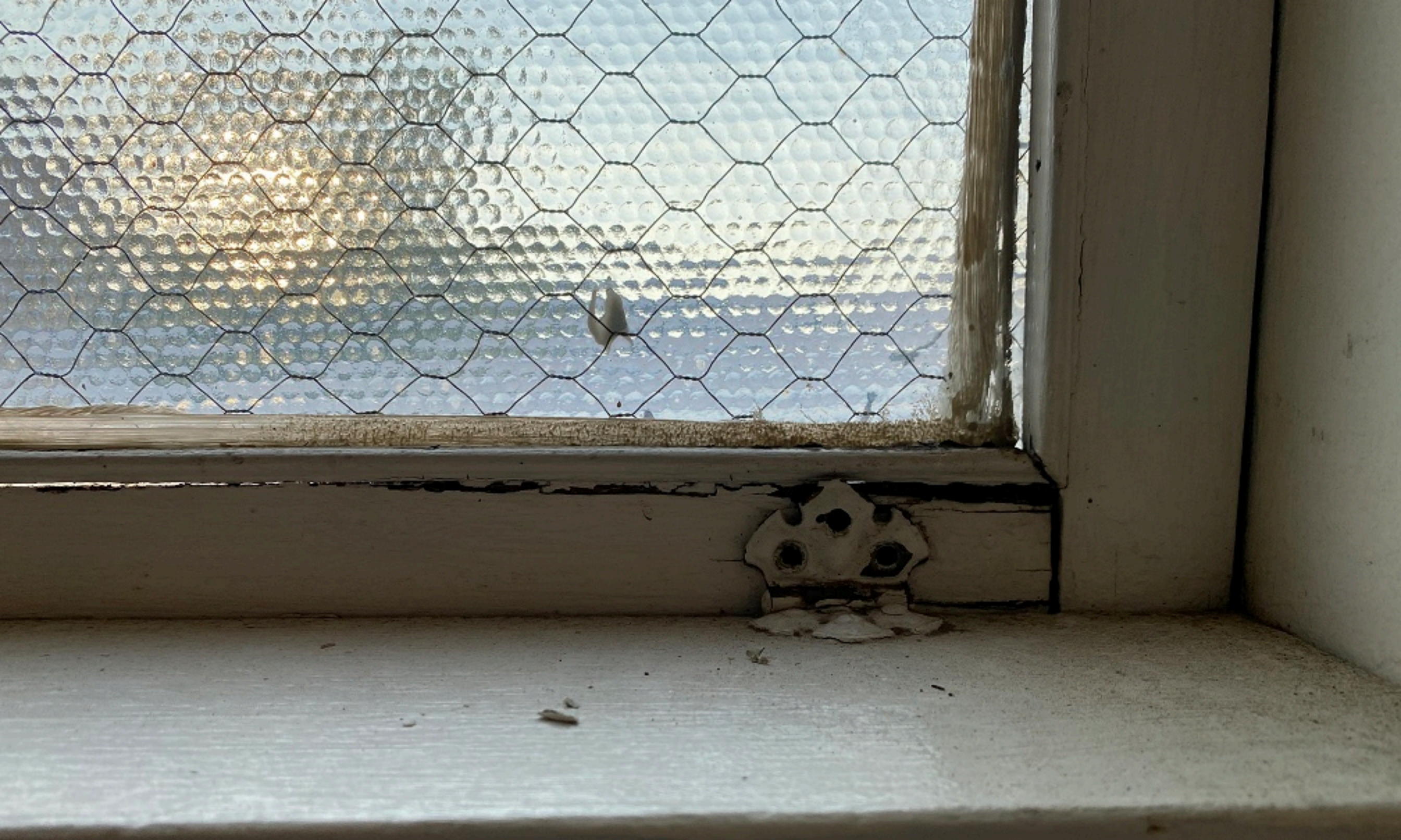
26.0 Deteriorated Bottom Rail at Window E and Damaged Wood Glazing Stop at Window E
