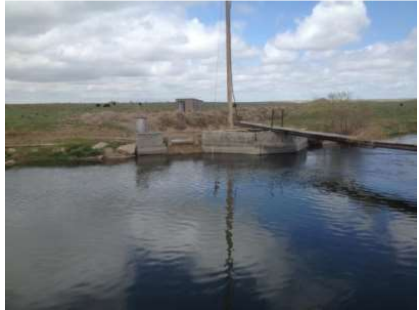
Riverside Diversion which feeds the Rothe/Sublette Recharge Project
