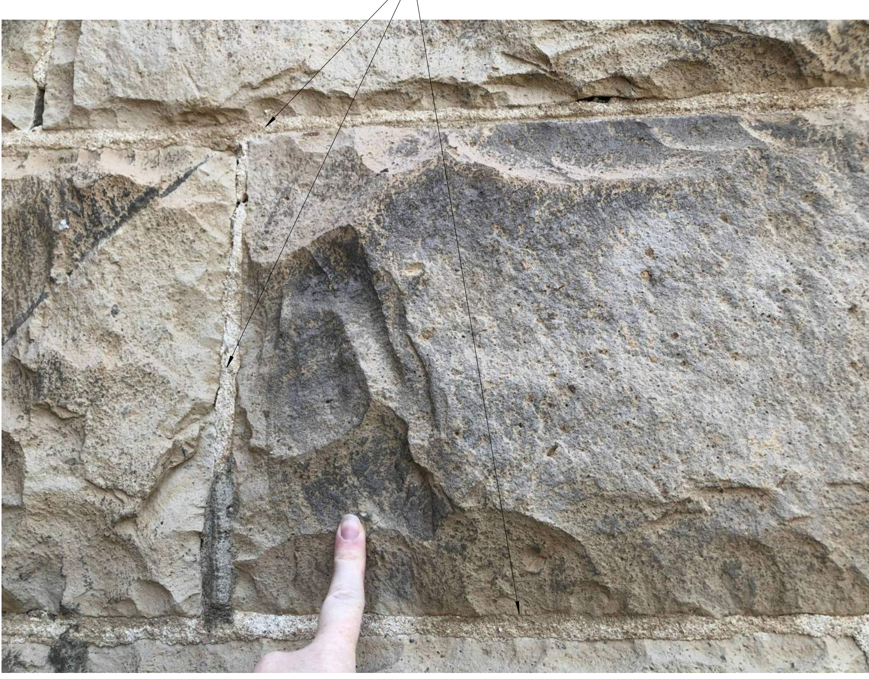
A4 EXAMPLE OF INAPPROPRIATE MORTAR NTS
