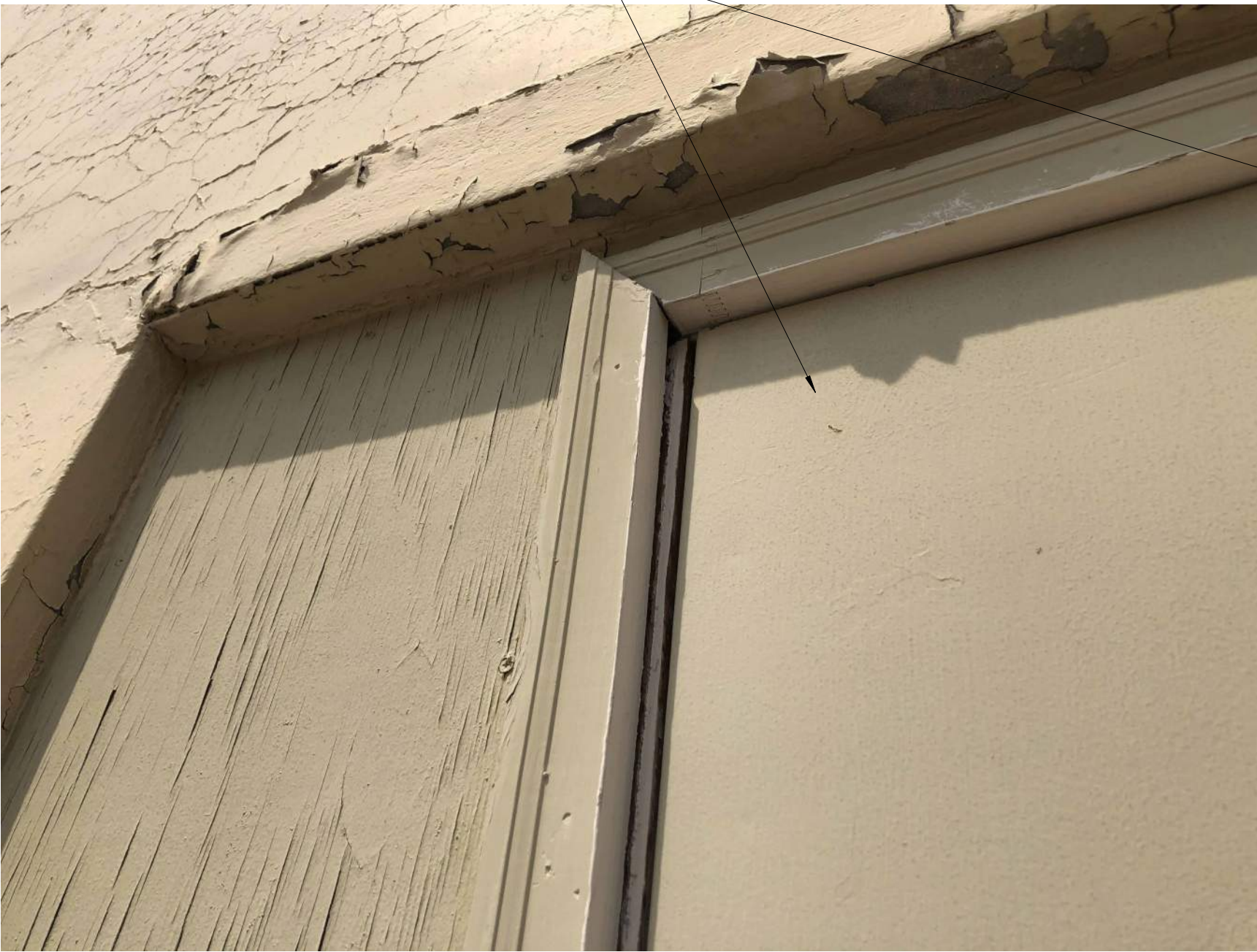
B4 DAMAGED STUCCO NTS
