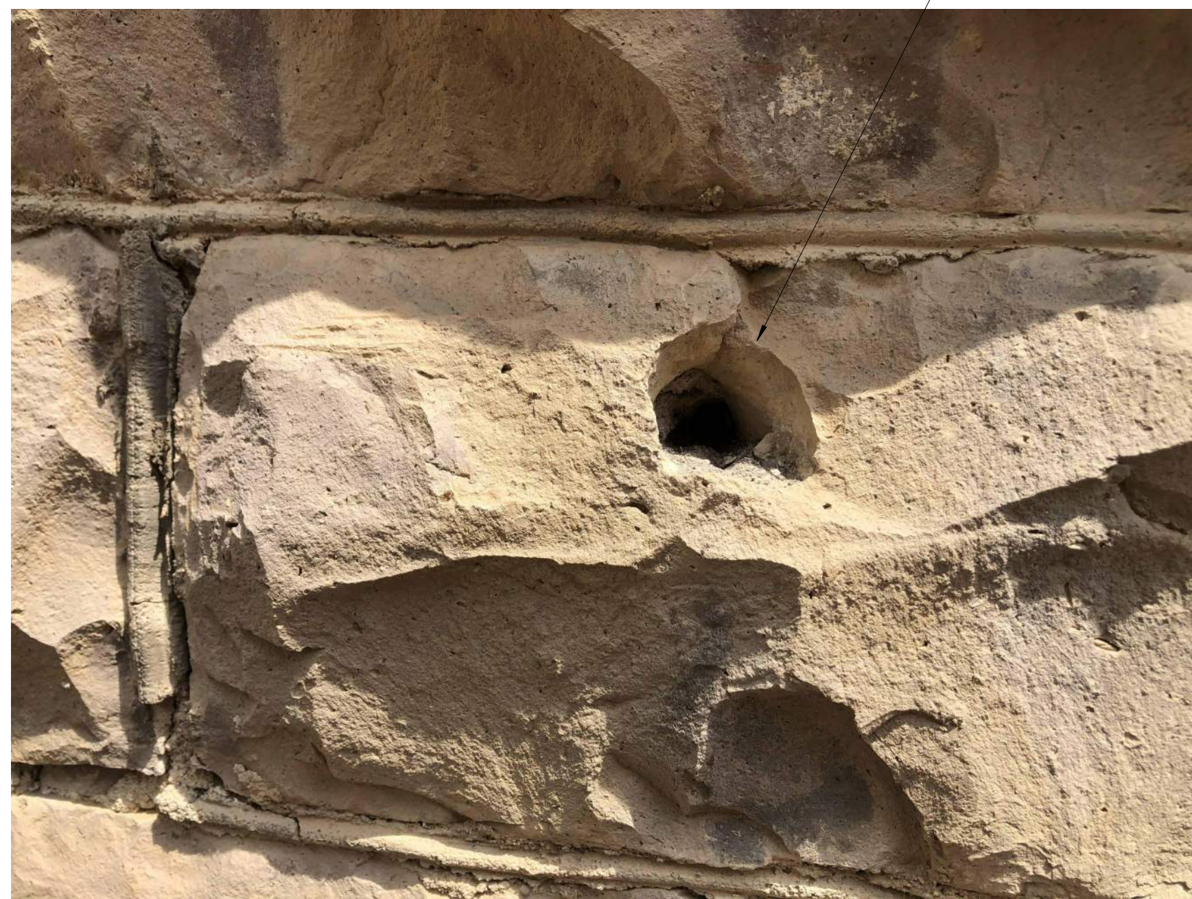
D1 EXAMPLE HOLES IN STONE NTS
