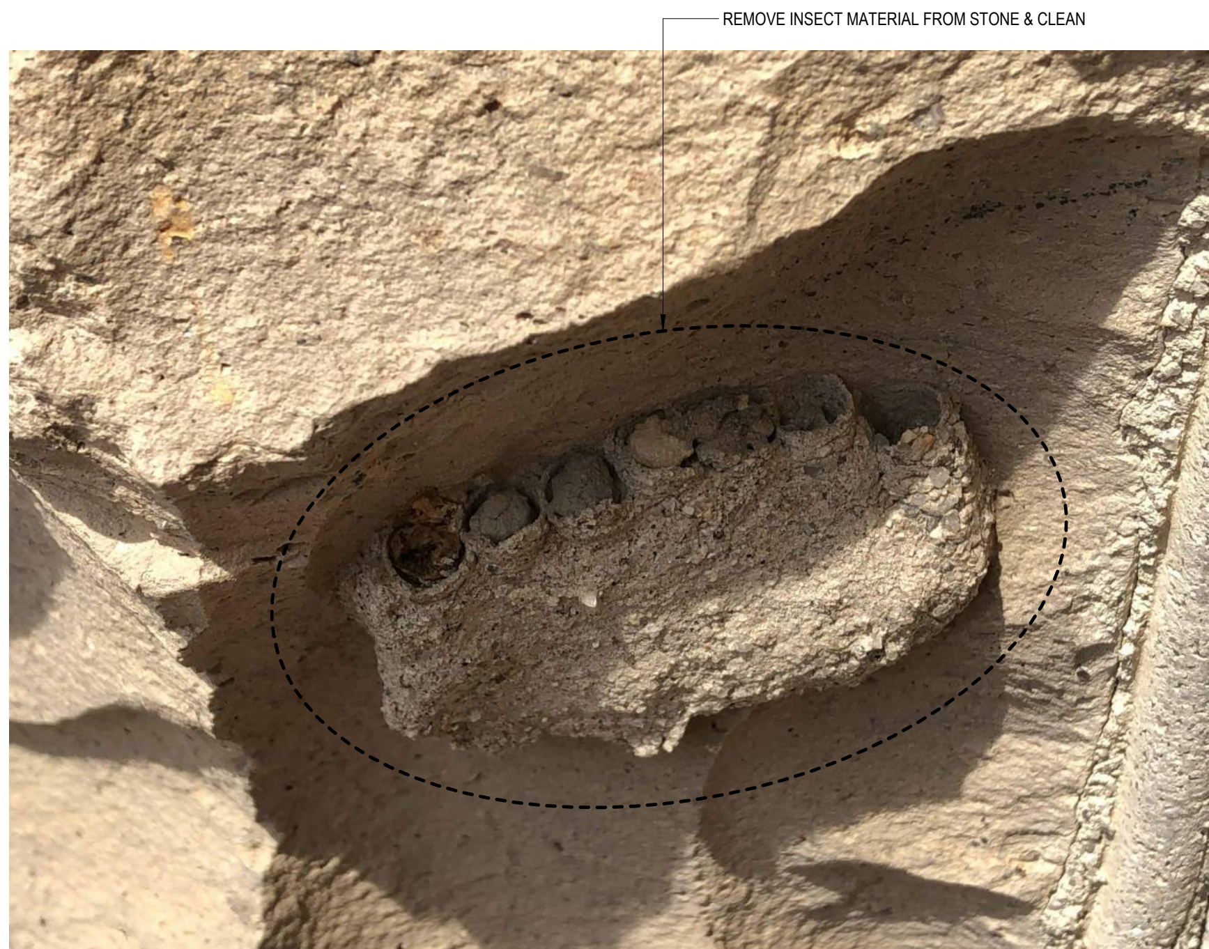
A6 REMOVE ORGANIC MATTER FROM STONE NTS
