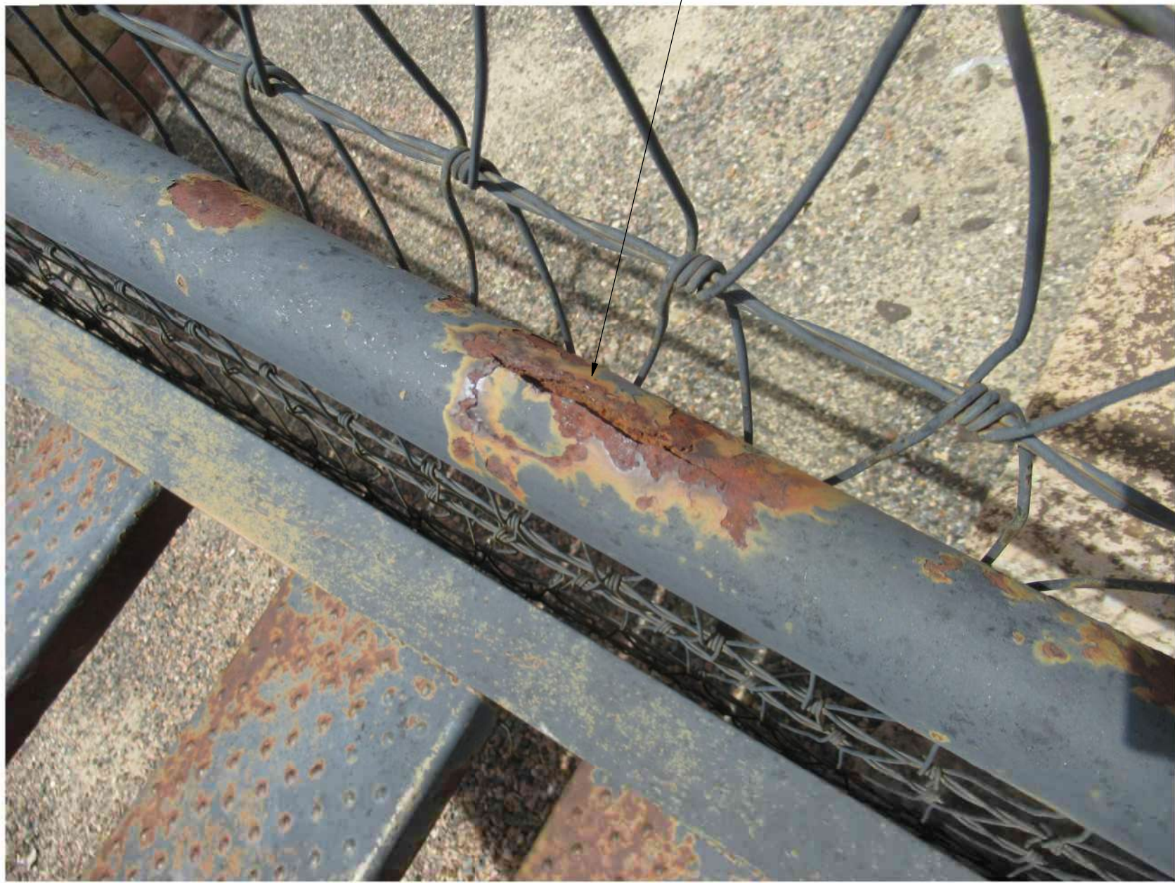
5 EAST FIRE ESCAPE RAIL - RUSTED S501 NO SCALE
