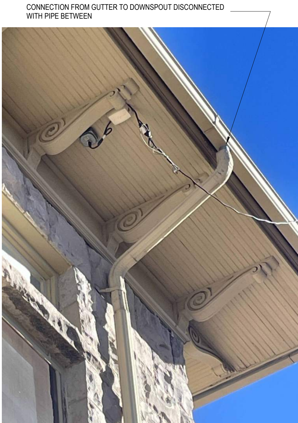
D3 DISCONNECTION AT DOWNSPOUT NTS
