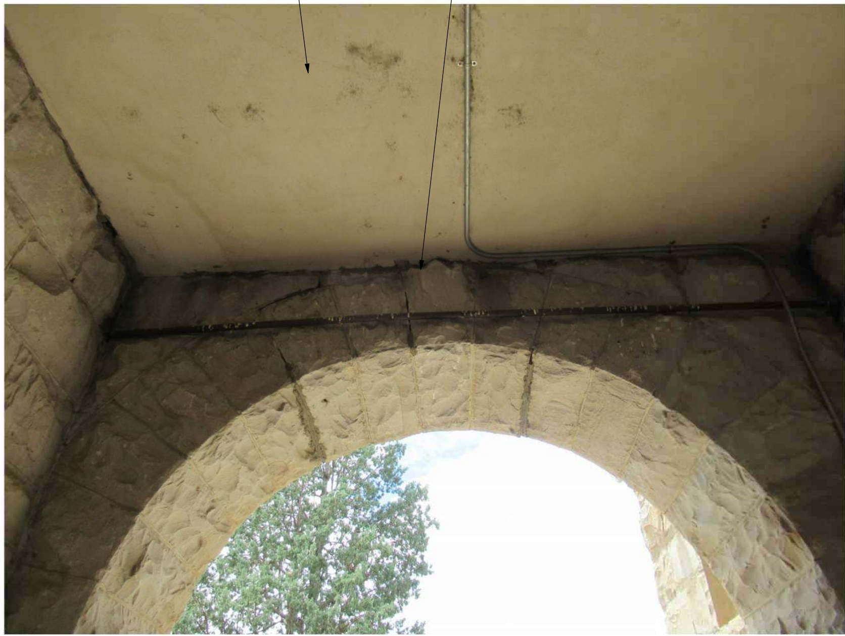
2 DROPPED ARCH AT TOWER ENTRY, WEST ELEVATION S501 NO SCALE
