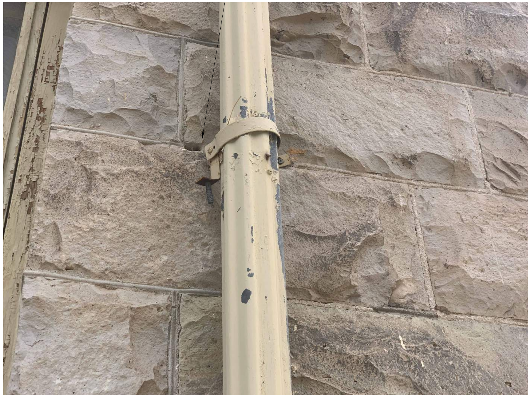
A1 DOWNSPOUT ATTACHMENT POINT NTS
