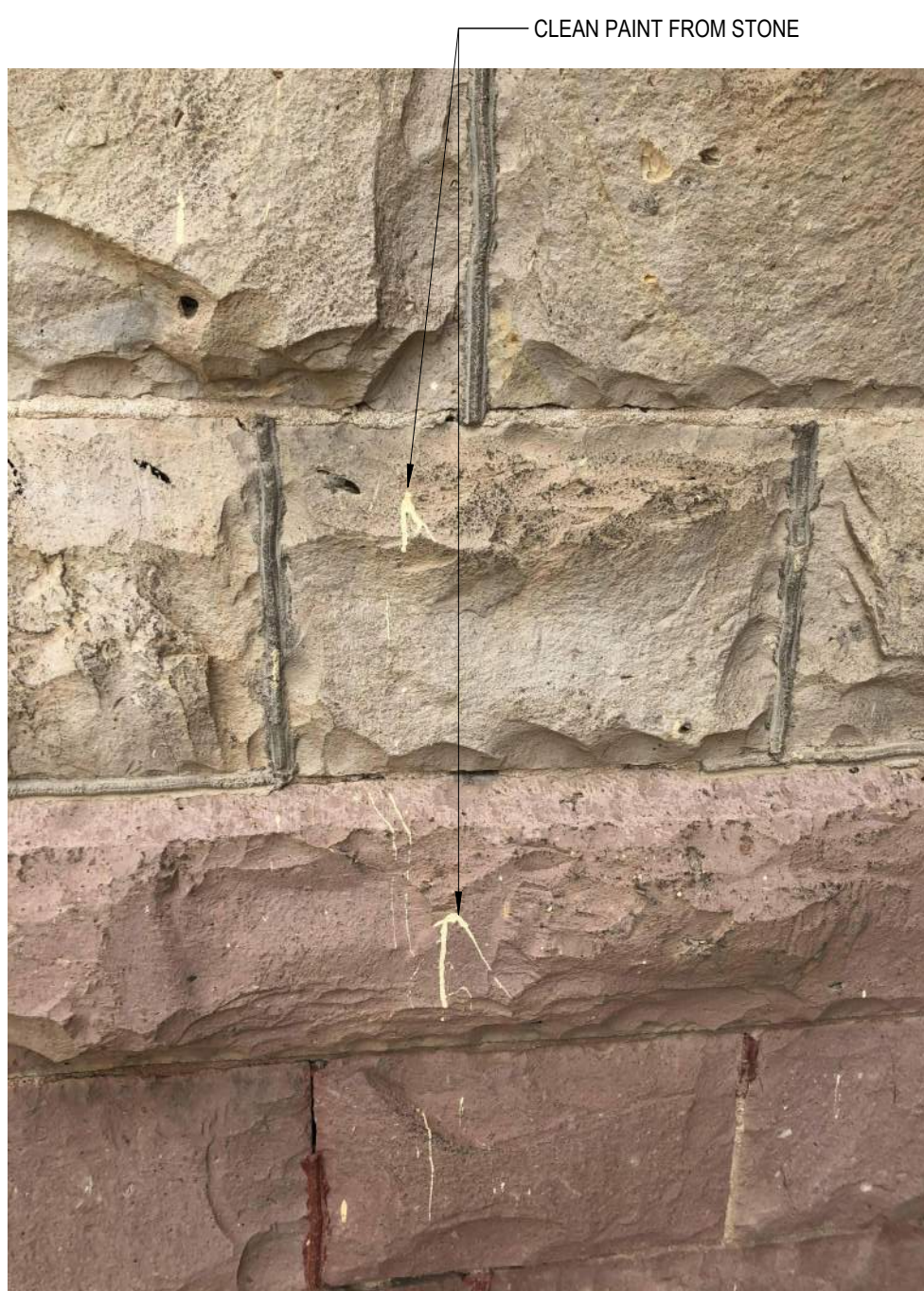
A5 REMOVE PAINT FROM STONE NTS
