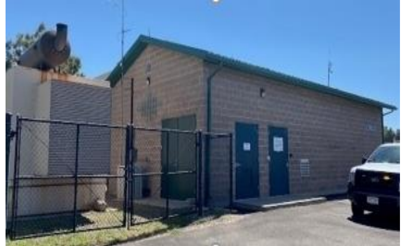
Pump Station Site
