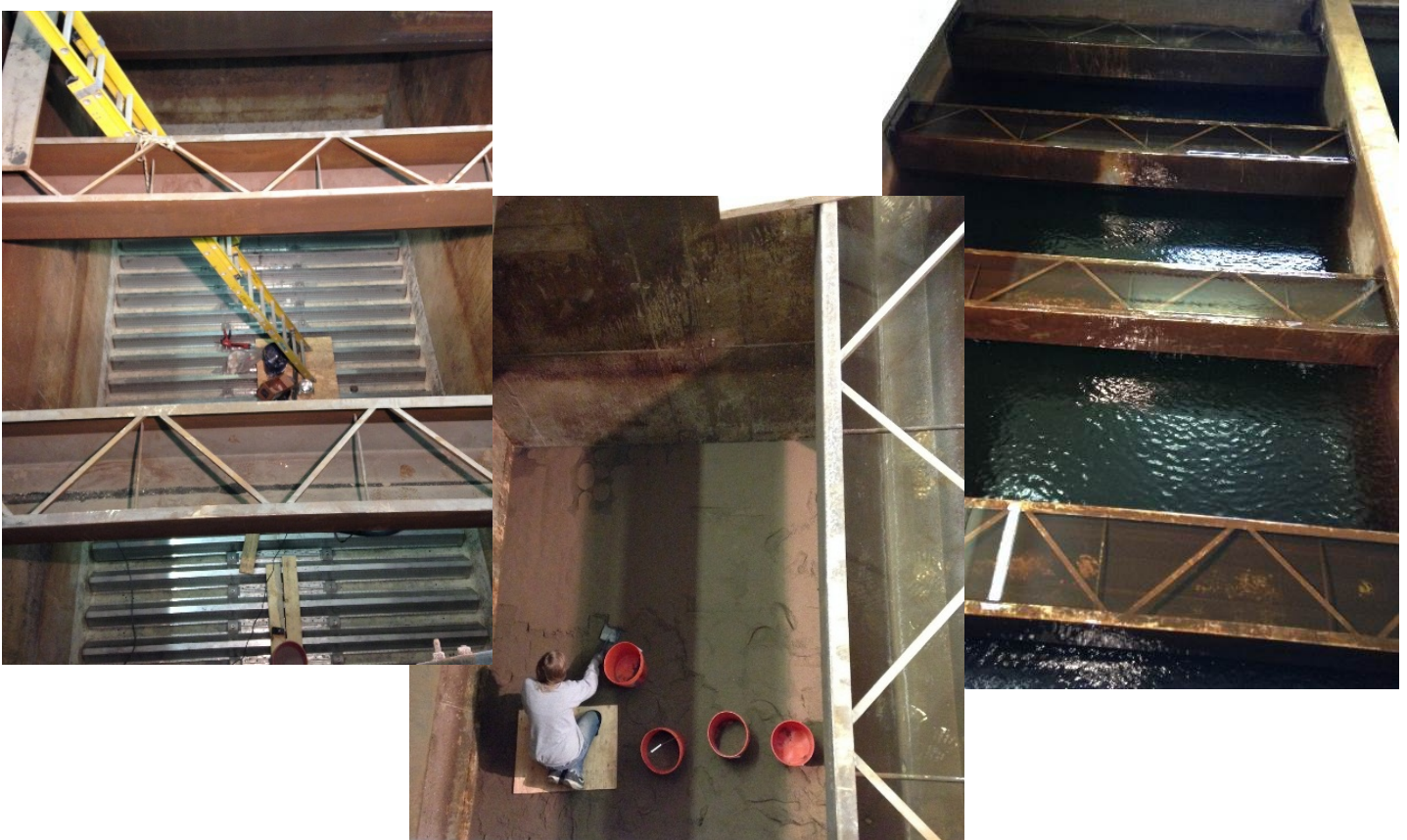
Showing stages – new underdrains installed, skimming fines off media layers during installation, and filtering water after completion.
