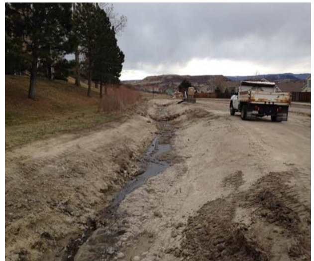
Plum Creek Ditch After
