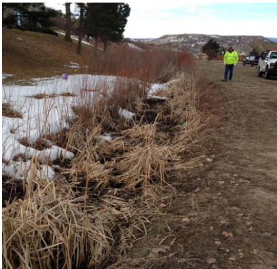
Plum Creek Ditch Before
