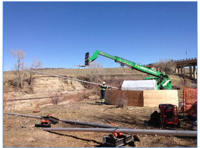
AL-16 lateral arm installation.
