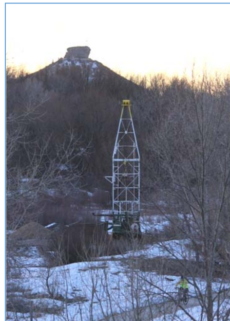
AL-18 vertical well drilling.
