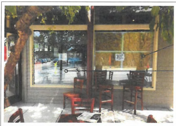
Existing Windows (from Perry St)
