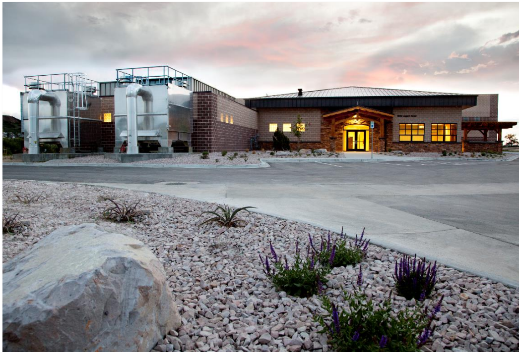
Plum Creek Water Purification Facility
