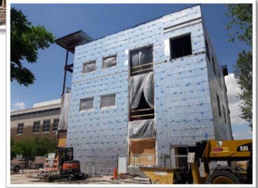
Town Hall Addition - June 30, 2017
