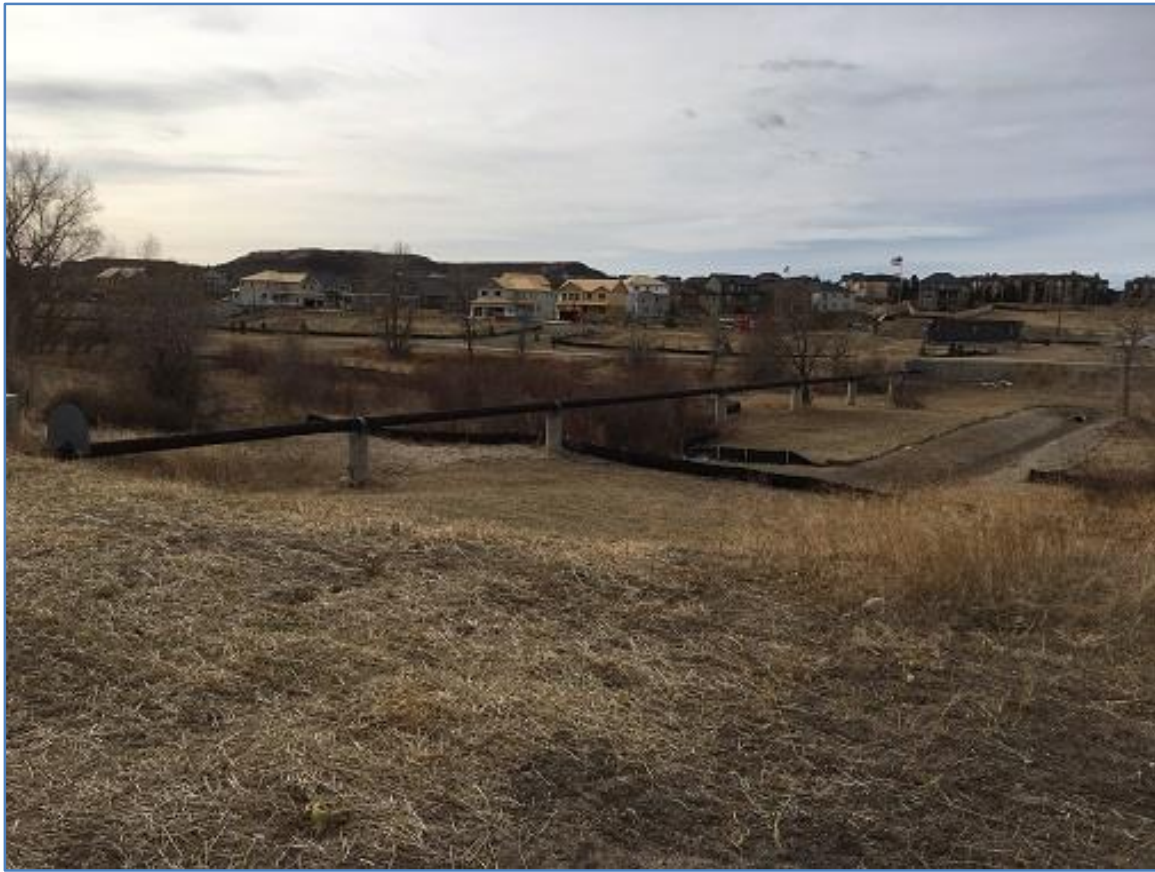
Elevated sewer over Sellars Creek at Gilbert Street. An elevated sewer was preferred to a lift station to serve a small area.
