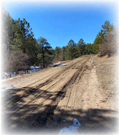
A significant amount of rutting in the road can be observed after use, especially after a storm.
