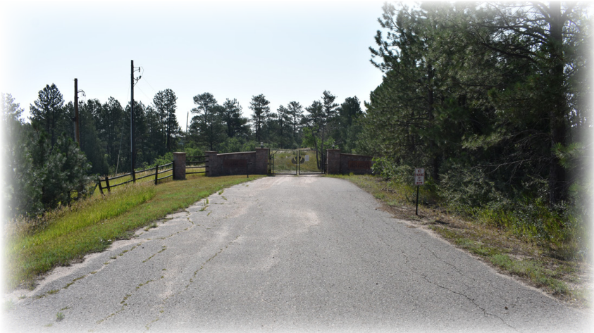
Asphalt at the main entry is deteriorating and breaking away at the edges.
