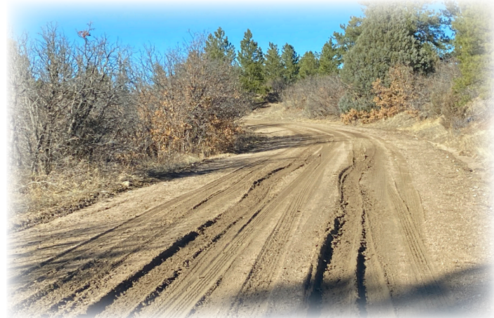
A significant amount of rutting in the road can be observed after use, especially after a storm.
