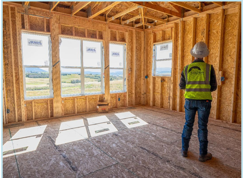
Site inspection performed by a Development Services Building Inspector.
