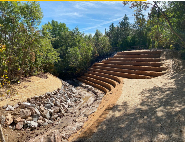
Stream stabilization (above) was done on an area along a trail with erosion issues (below) that had been identified by a resident.
