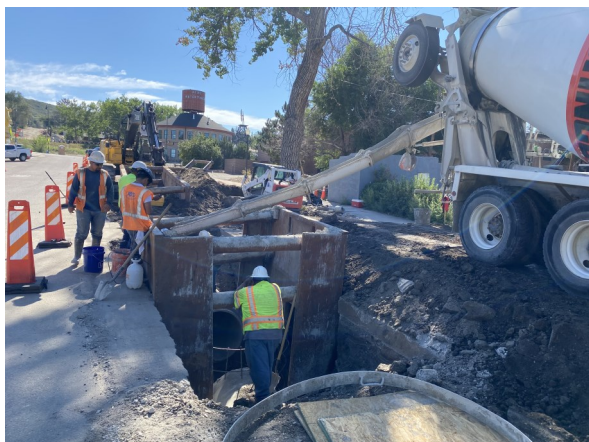
Storm sewer outfall, water main and sewer main in Sixth Street.
