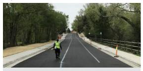
Client Reference Brent Thompson, PE City of Littleton P: 303-795-3798 Benesch provided preliminary and final design services for a reconstructed section of Bemis Street. Benesch's design created a continuous and ADA compliant sidewalk connection, installed curb ramps, addressed drainage issues and clarified parking lane locations.
