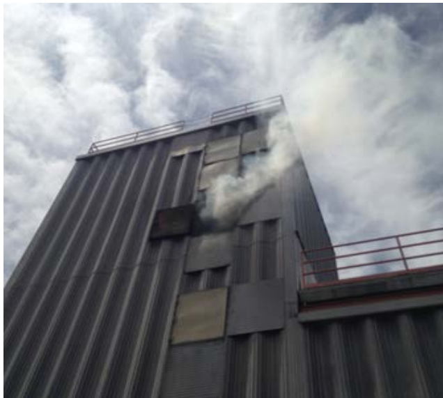
Smoke showing on the 4 th floor
