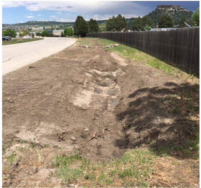
The Stormwater Team removed a tree and regraded the roadside ditch to re-establish a proper drainage channel along Topeka Way.
