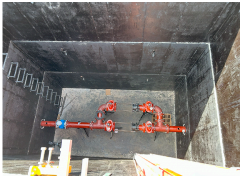
The interior of the vault.
