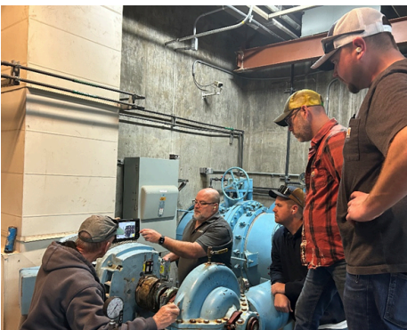
Training for Ops on a new laser alignment tool, which is designed to align shaft motors.
