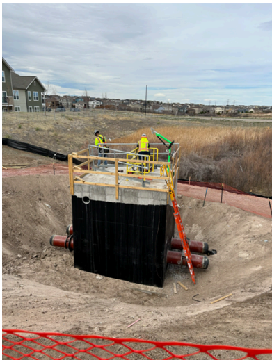
New 20-inch steel lines and excavation. March 2026
