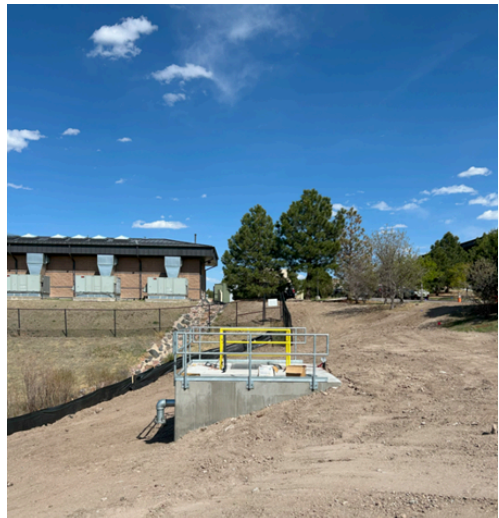
Backfill and rough grading around the vault completed. April 2026
