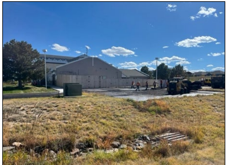
Driveway repair Station 154
