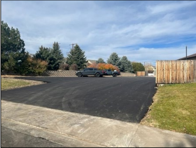
Driveway repair Station 153
