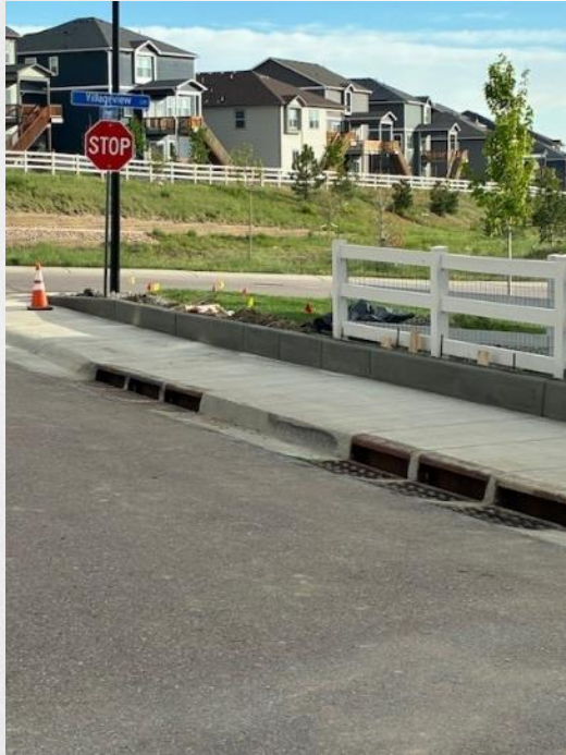
Overtopping stormwater inlets and lack of emergency overflow path
