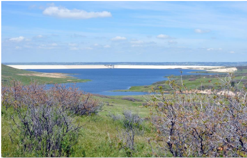
Looking northeast across Rueter-Hess Reservoir
