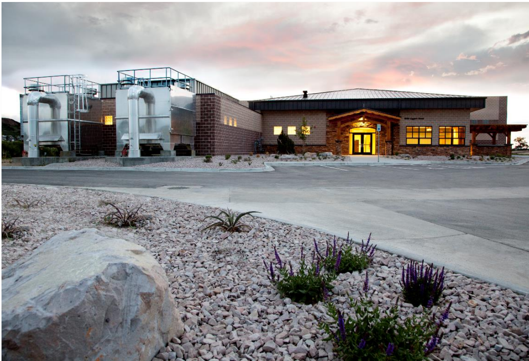
Plum Creek Water Purification Facility
