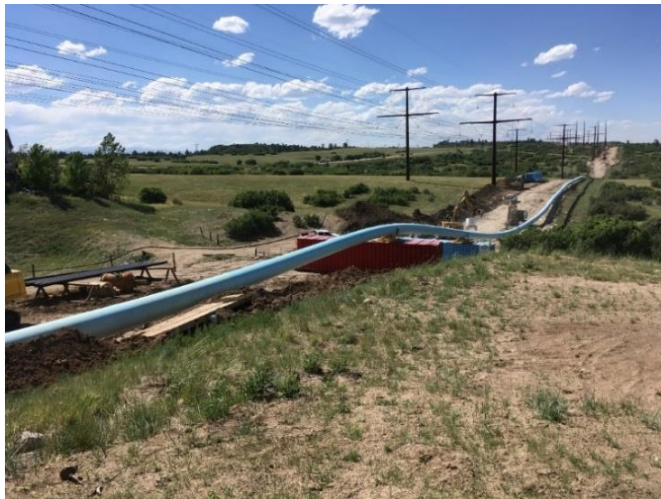
Wise Pipeline during Construction
