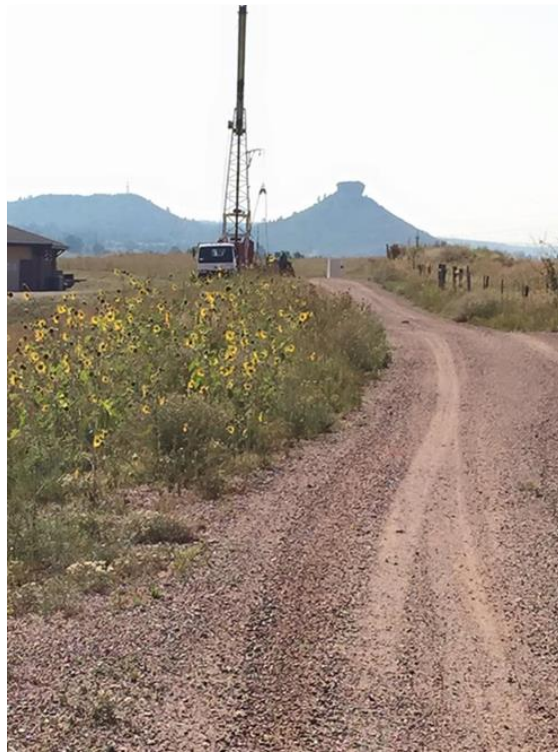
Well 223 undergoing maintenance activities
