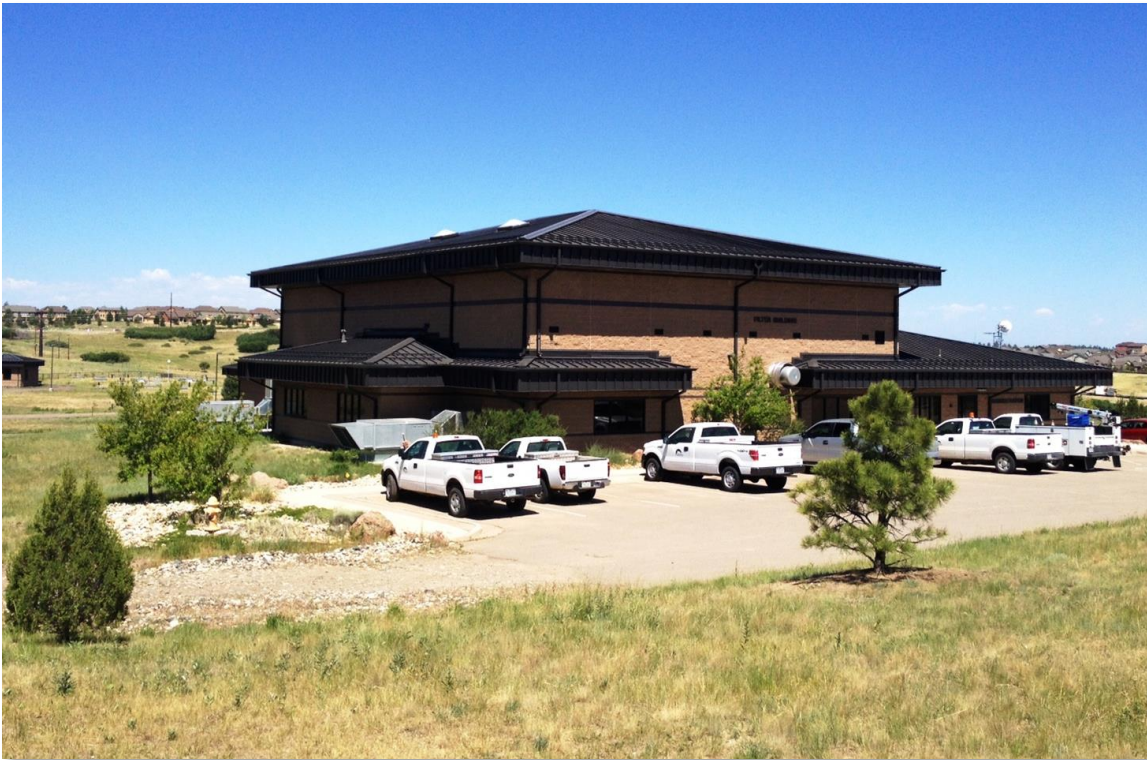
Ray Waterman Treatment Plant
