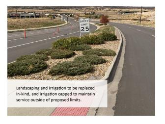
Roundabout enables us to apply similar water quality approaches for this project. Peakview/ Peoria incorporated bioswales into the newly created open areas between intersection legs. Underdrains in the bioswales were connected to adjacent inlets and conveyed in the downstream drainage system. The designs of water quality features and the release of flows to the existing drainage system would follow the guidelines of the SDDTCM.
