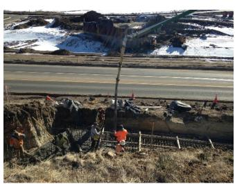
In early January weather was favorable to allow the contractor to construct foundation forms, place rebar mats and pour 95 cubic yards of concrete to complete abutment and wall footings. Additionally, three quarters of the abutments and wing walls have been constructed totaling an additional 80 cubic yards of concrete. The project is currently on schedule to be completed with the Philip S. Miller Park Phase two improvements this spring pending good weather conditions.
