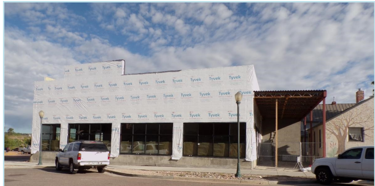
Photo of the Sushi Restaurant under construction at 301 Jerry Street.
