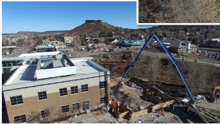
Above and Left: Foundation Wall Concrete Pour of March 2
