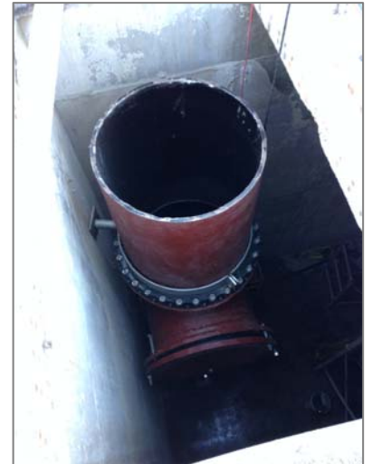
Left to right: Cutting and removing the 20,000 plus pounds of concrete, reinforcing and formwork for new concrete beam and hatch curb walls, and the new 42" diameter ductile iron pipe system.
