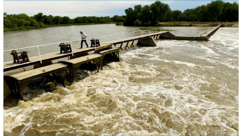
Diversion structure along the lower South Platte River in Northeast Colorado
