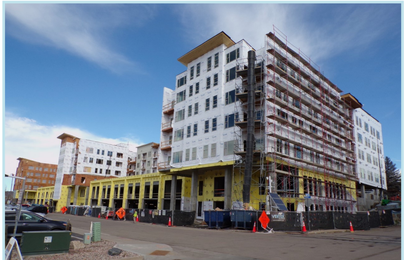
Construction of The View located at 205 Sixth St.
