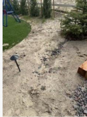
Yard damage in Crystal Valley Ranch
