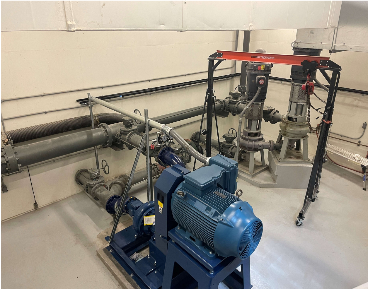
Castle Oaks Lift Station - New pump installation
