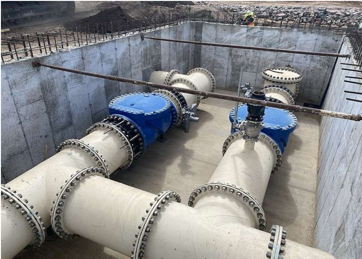
Castle rock Reservoir #2: Vault and new piping
