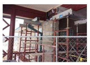
Over the past year, cracks emerged under two of the primary columns that support steel beams at the Metzler Restroom and Concession building. For the past several months, a structural engineer and contractor have developed solutions for the issue and repair work began in late November. Repairs will be complete by the second week in December.
